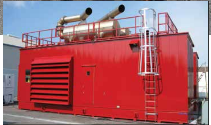
This red enclosure is a 2500KW drive unit for a crane. This enclosure also has an extremely specialized interior.
